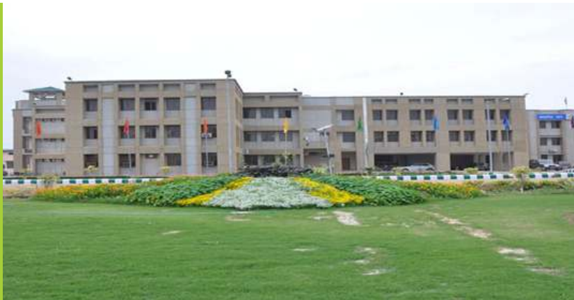
Administrative Building SJUA&T, MEERUT
